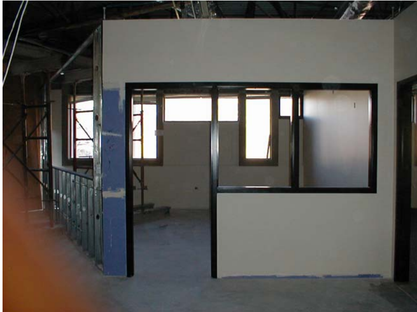
New offices on the 600 level
