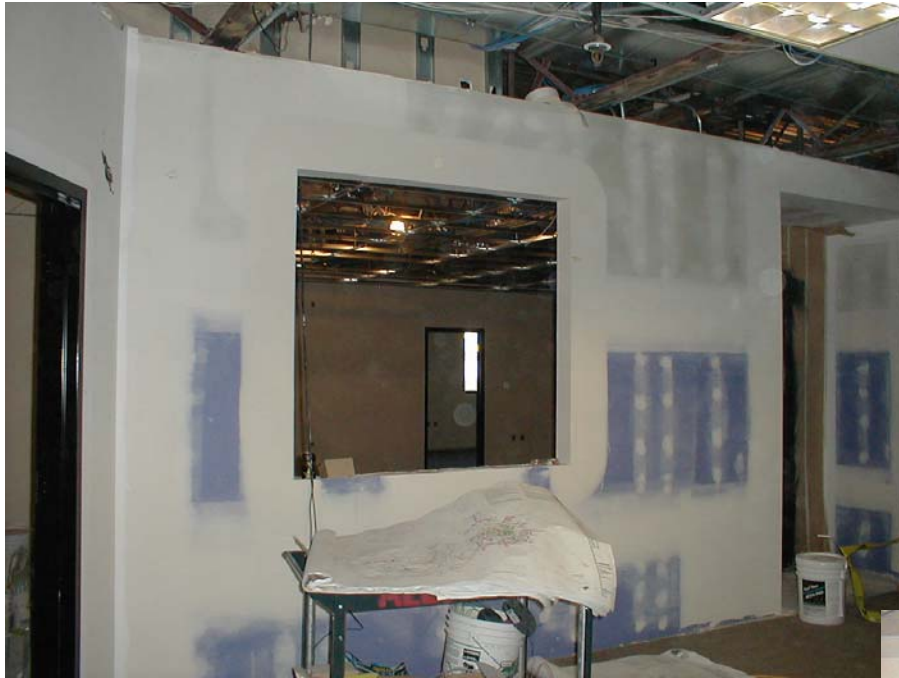
New attendance window on the 800 hallway.
